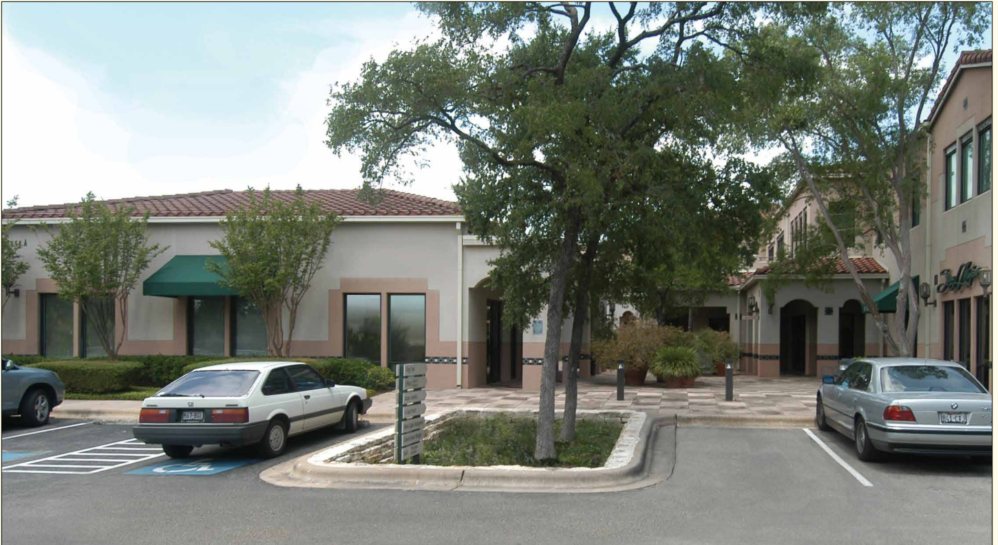
BUILDING 2·WEST TO THE LEFT
